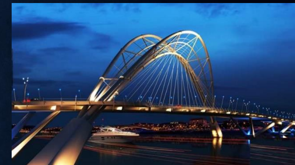
Ben Nghe Bridge (Thu Thiem 4)
