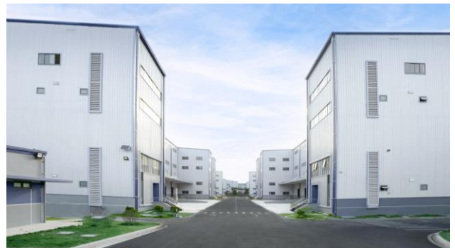
Exhibit 20: BW Nhon Trach 1 – a pioneering double-story RBF facility in Vietnam
